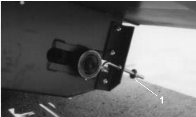
Figure 20 Conveyor Tail Pulley
